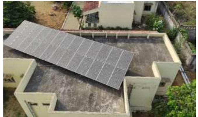
**Solar panels installed for water pumping**
